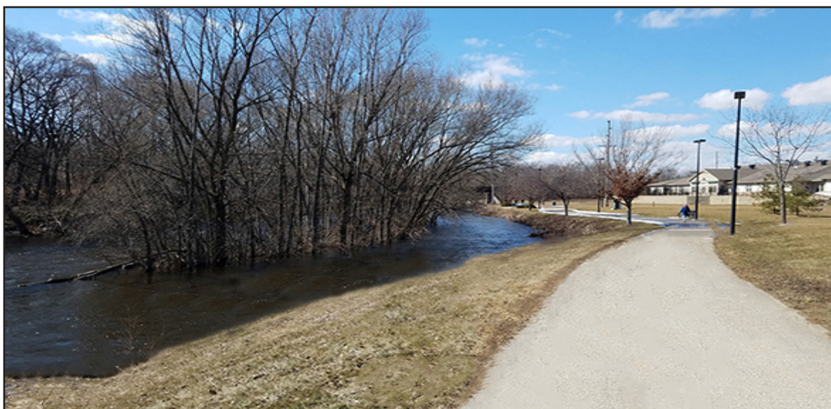
Shared Use Path Riverside Park Trail along the Milwaukee River in the City of West Bend
